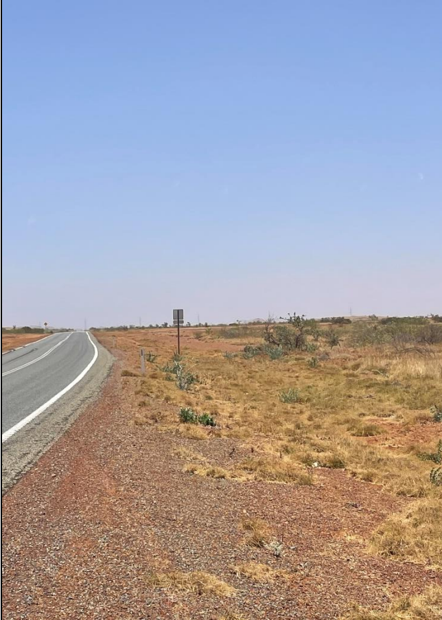
Photo 3. Looking South along North West Coastal Highway on the northern side of the road at SLK 1095 - Photo taken 25/11/2023
