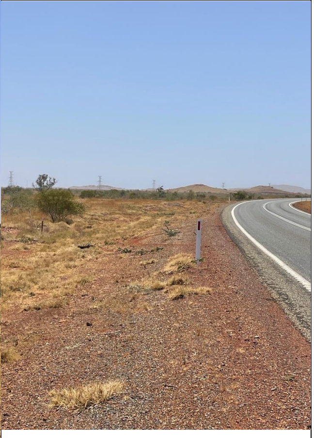
Photo 4. Looking South along North West Coastal Highway on the northern side of the road at SLK 1095 - Photo taken 25/11/2023
